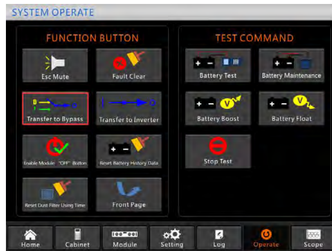
The operation interface for transferring to bypass
