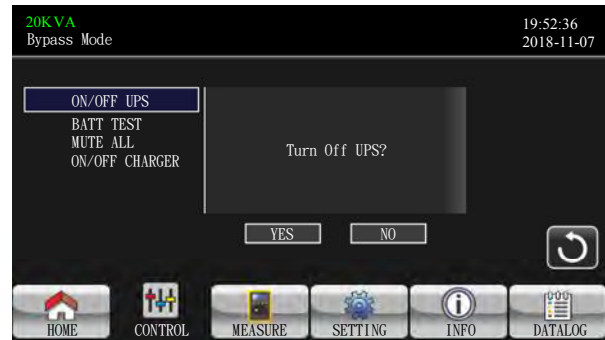
TURN OFF UPS
