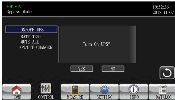
TURN ON UPS
